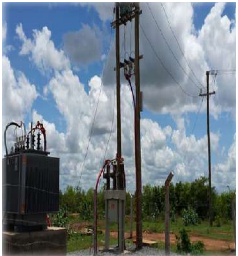
Installation of transformer 315kVA and cable termination at Geita.
