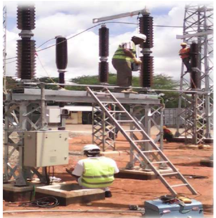
Testing and commissioning of 220kV reactor at Singida switchyard.
