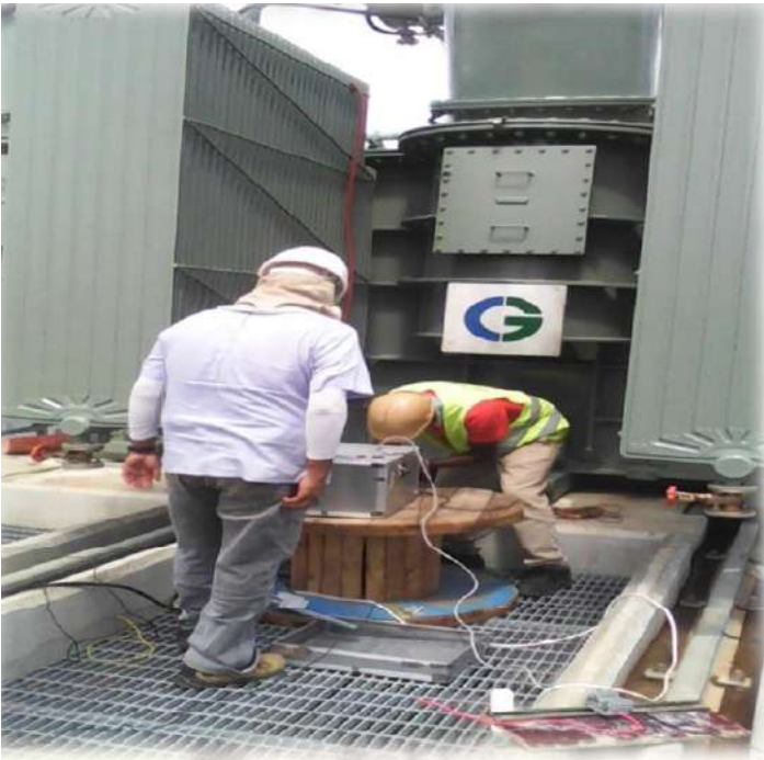
Testing and commissioning of 220kV reactor at Singida switchyard.
