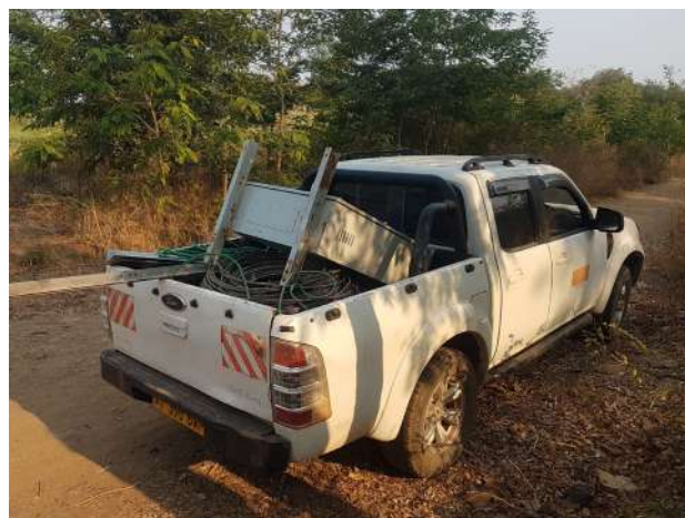
Installation of power house, step-up transformer and back up generator in Kigoma
