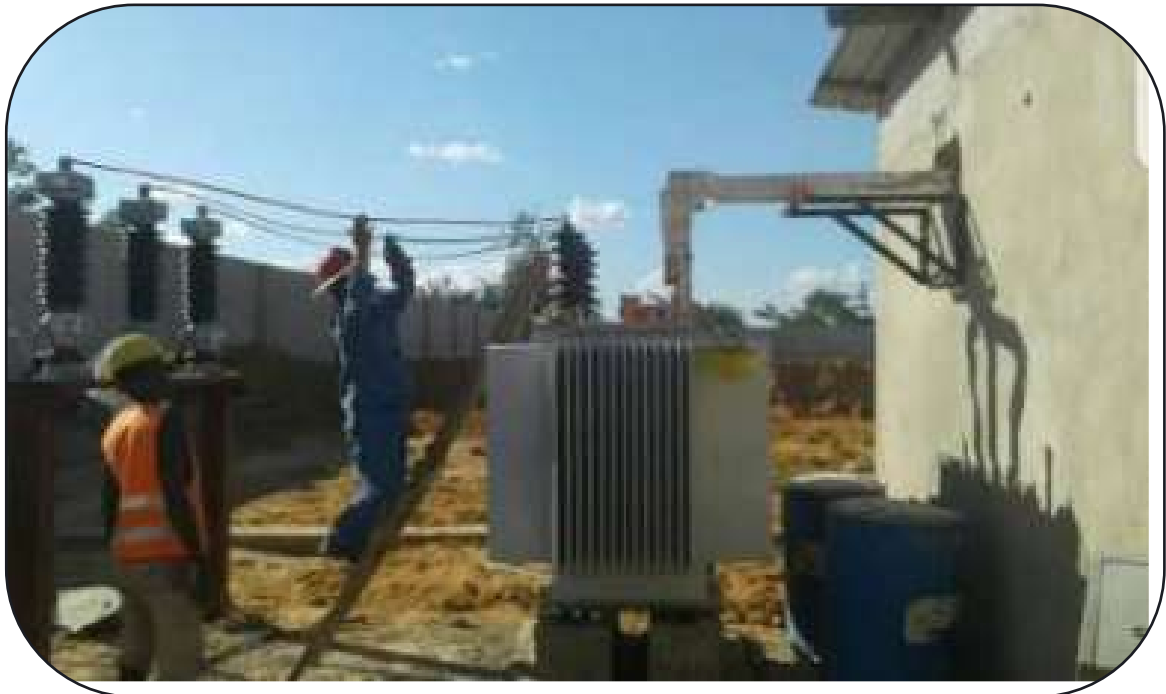
Installation and commission of transformer (800kVA) and power factor at Sayona steel, Mwanza.
